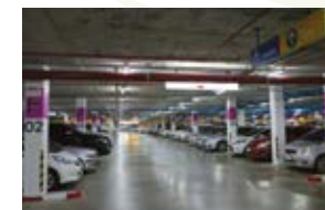
Underground car parks
